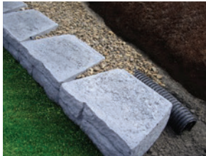
5. Lay drain coil and drainage aggregate
