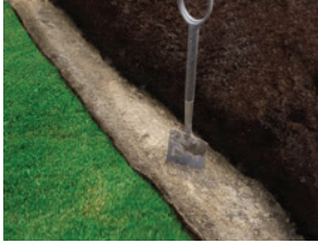
1. Mark out and dig trench
