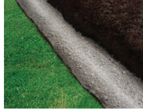
2. Fill trench with WESTSTONE-BASE-COURSE
