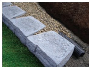
5. Lay drain coil and drainage aggregate
