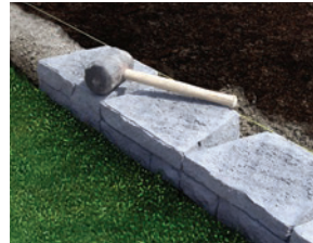
4. Lay first layer
