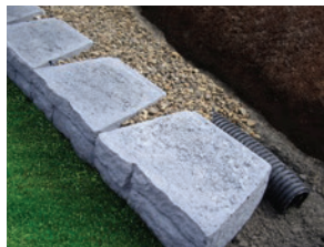
5. Lay drain coil and drainage aggregate
