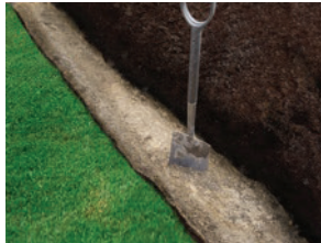
1. Mark out and dig trench
