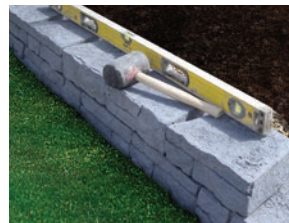
6. Lay second layer, continue laying and check levels
